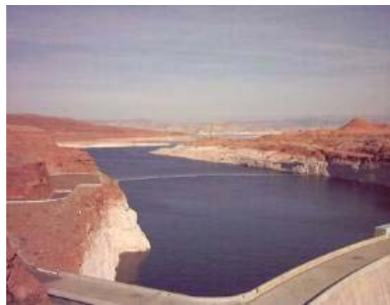
FIGURE 11.1.2 Lake Powell reached a record low level of 3555 feet MSL in April, 2005, over 105 feet below normal and corresponding to less than 50% of normal storage. By September 26, 2006 the water level had recovered to 3602 feet MSL.
