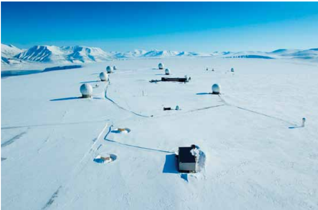
NASA's downlink facility in Svalbard, Norway located at 78° North latitude. This is an ideal site for receiving data from polar-orbiting satellites like Aura, because these satellites pass within range of the station on every orbit.
