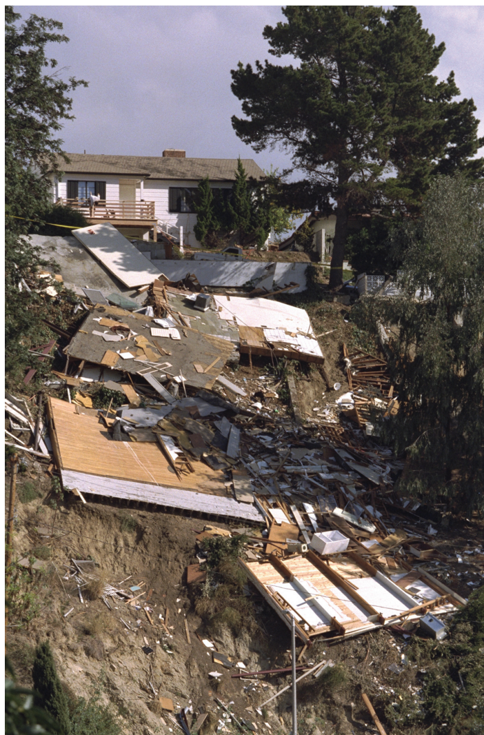
FIGURE 8.5 Earthquakes produce substantial economic and human loss that could be mitigated with better warnings. In the Northridge, California, earthquake of January 17, 1994, buildings, cars and personal property were all destroyed when the earthquake struck. Approximately 114,000 residential and commercial structures were damaged and 72 deaths were attributed to the earthquake. The cost of damage was estimated at $44 billion (NRC, 1999). SOURCE: FEMA News Photo.
